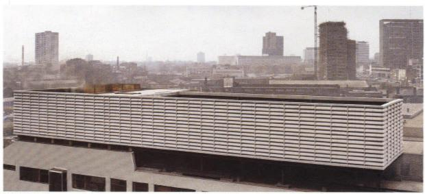
Noishield® Louver cooling tower inlet screen/noise barrier. Note how "clean" lines, color, and mitered corners provide attractive, uncluttered appearance architecturally compatible with the surroundings.
