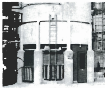
STRUCTURES WITH SILENCERS Furnace Noise Reduction 23 dBA
